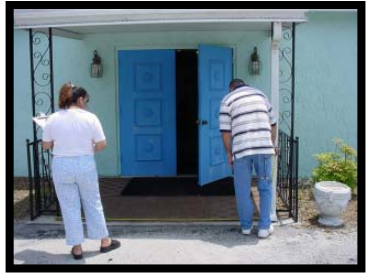
The degree of slope in the parking lots, walkways, and ramps leading into the facilities were measured with the ADA Accessibility Stick.
